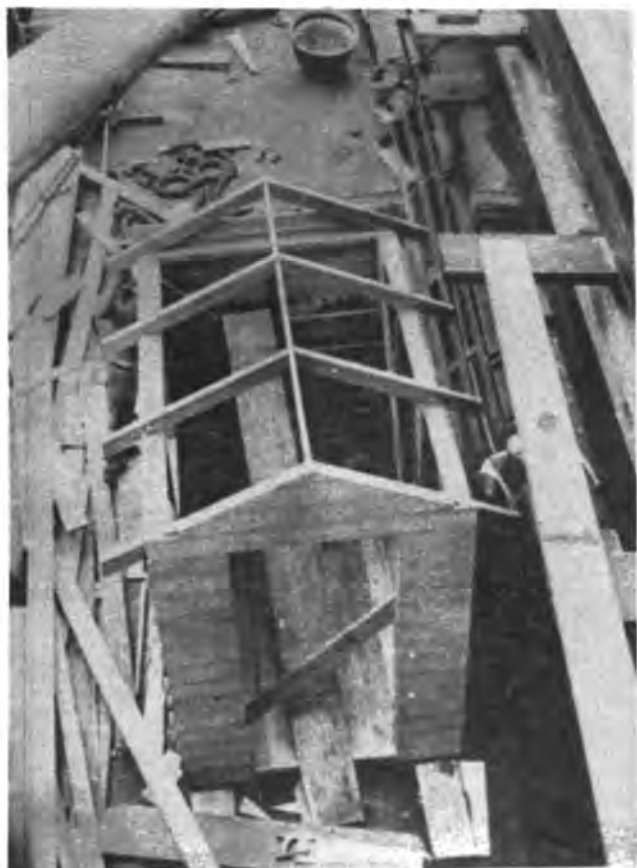
Temporary radio shack destined for Wake Island stowed aboard the SS North Haven (KUDZ) in April 1935 en route with material and equipment with personnel to establish and man the PAA bases at Midway, Wake, Guam and Manila. Pix taken by Capt. Almon A. "Al" Gray 810-P
